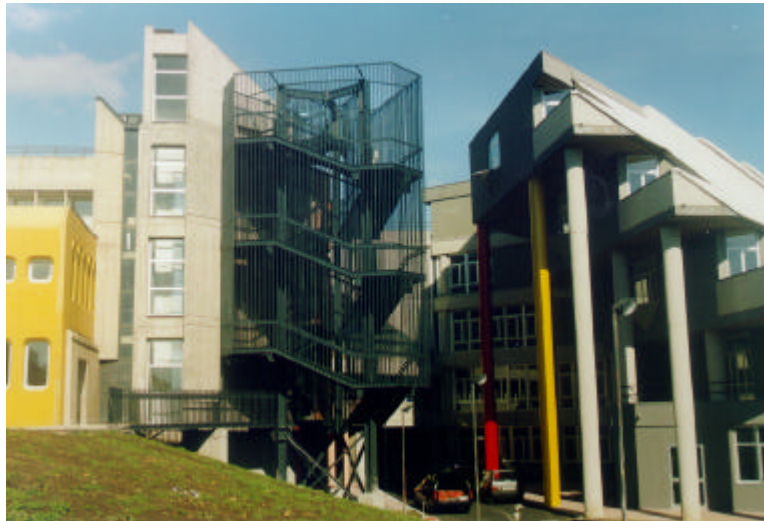
Fig. 1: Staircase under study
